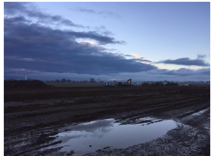
Weather day-no work completed (11/22)
