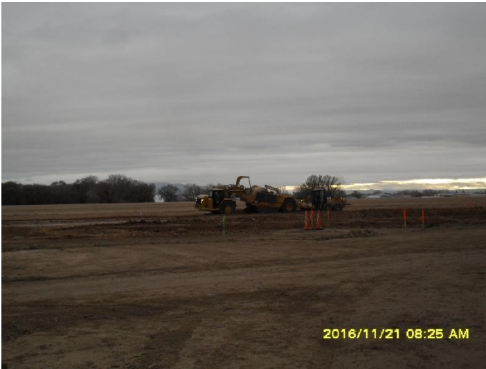
P-152 excavation to embankment and compaction (11/21)
