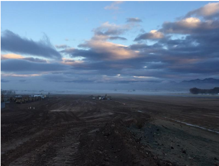
Weather day-no work completed (11/22)
