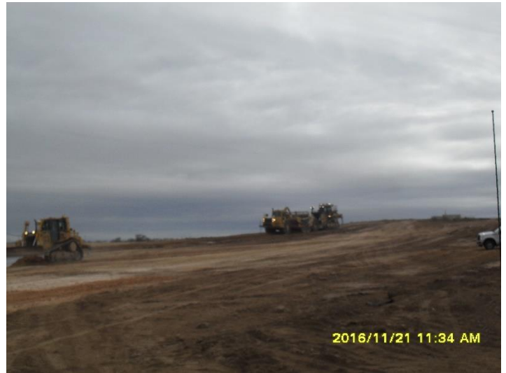
P-152 excavation to embankment and compaction (11/21)
