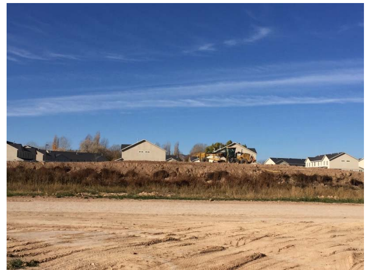
Blading topsoil piles (11/8)
