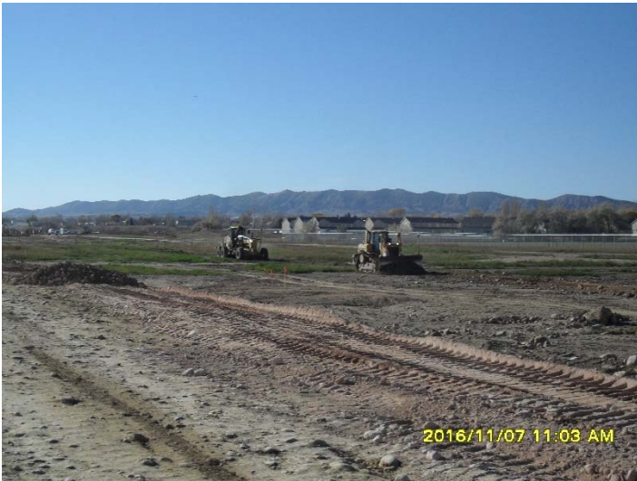
Establishing haul road (11/7)
