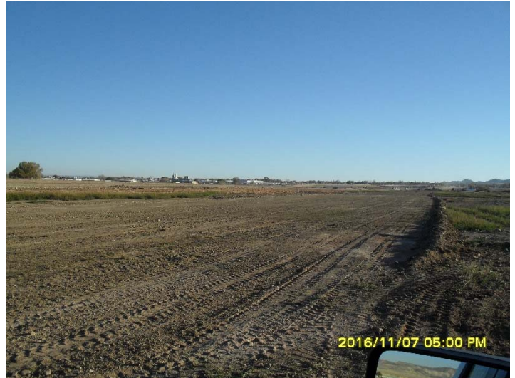
Establishing haul for scrapers for topsoil stripping (11/7)
