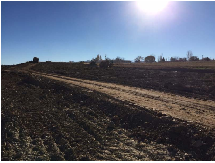
Stripping topsoil (11/10)
