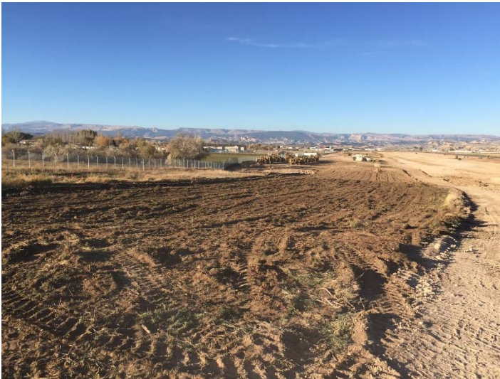
Establishing haul for scrapers for topsoil stripping (11/8)
