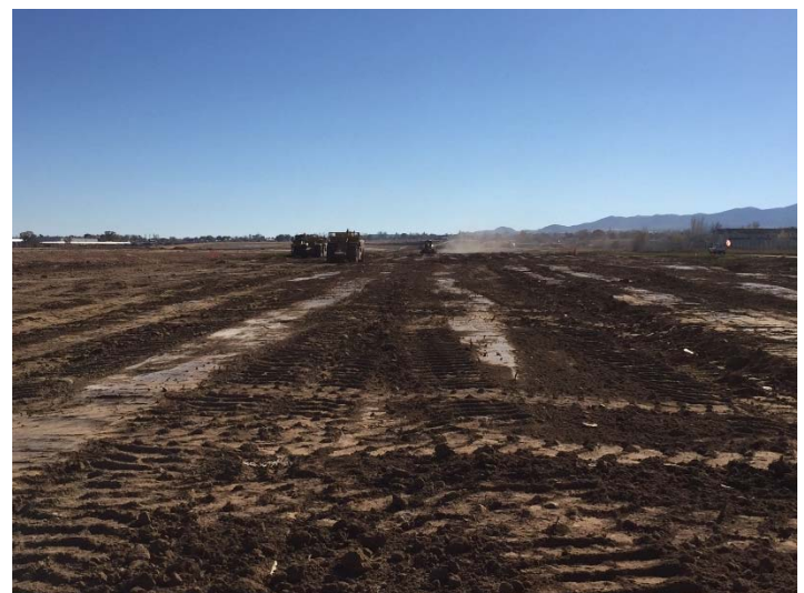
Stripping topsoil (11/9)
