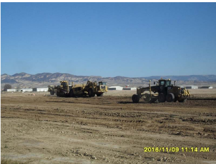
Stripping topsoil (11/9)
