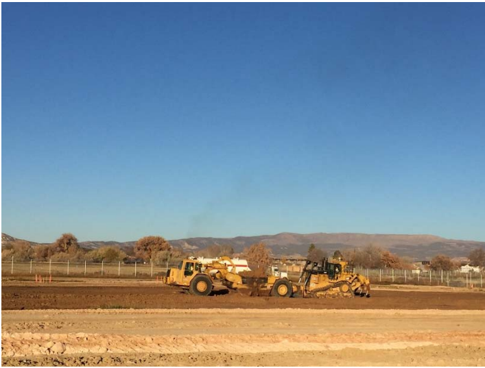
Stripping topsoil (11/10)
